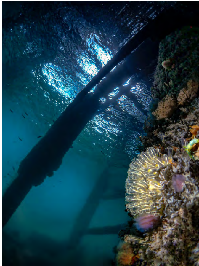
Life in those legs- from Swanage Pier looking up at the structure while capturing the life on the leg. Olympus TG4 -Weefine WFL-02 Light and Motion Gobe wide light- FNumber: 2.8, Focal Length: 4.5
