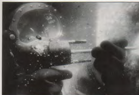
(Above) Commercial diver John "Legs" Diamond cuts a wharf pile in Napier Harbour, New Zealand. Diamond was the cutter in the H.M.S. Edinburgh salvage in the Barent Sea. Nikonos III with 15mm lens and single handheld wide-angle strobe on a very long arm. Visibility approximately 0.75 metres. Fujicolor 100 printed and then copied with reversal film Fujichrome 50.
